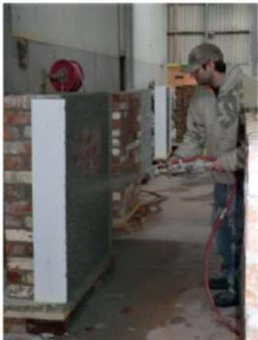
(b) Spraying of ECC shotcrete onto wallette
